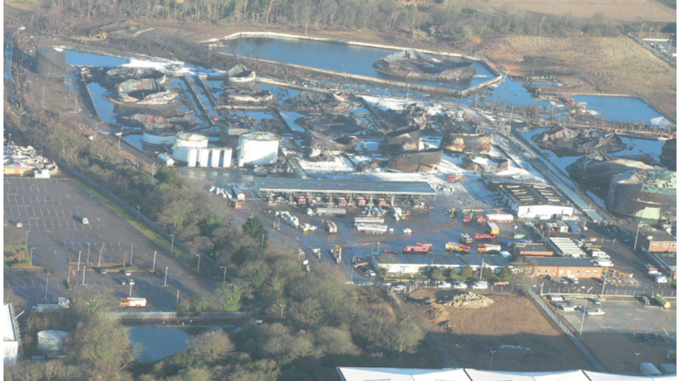
Figure 5 Part of the Buncefield depot after the incident © Chiltern Air Support
