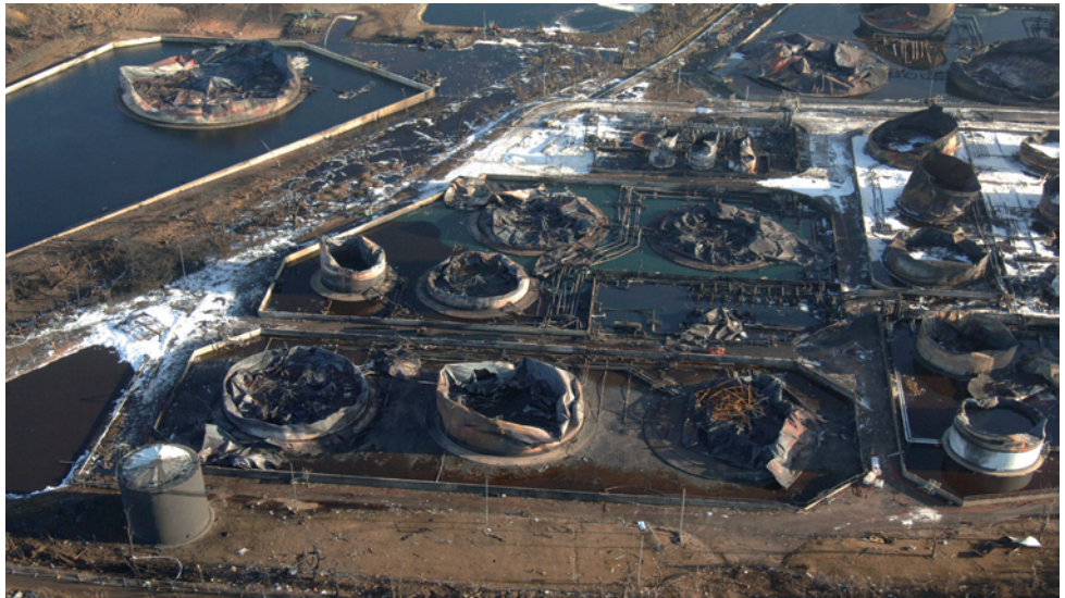
Figure 6 Buncefield after the incident: Tank 912 is in the centre foreground and Tank 12 is in the top left of the picture © Chiltern Air Support
